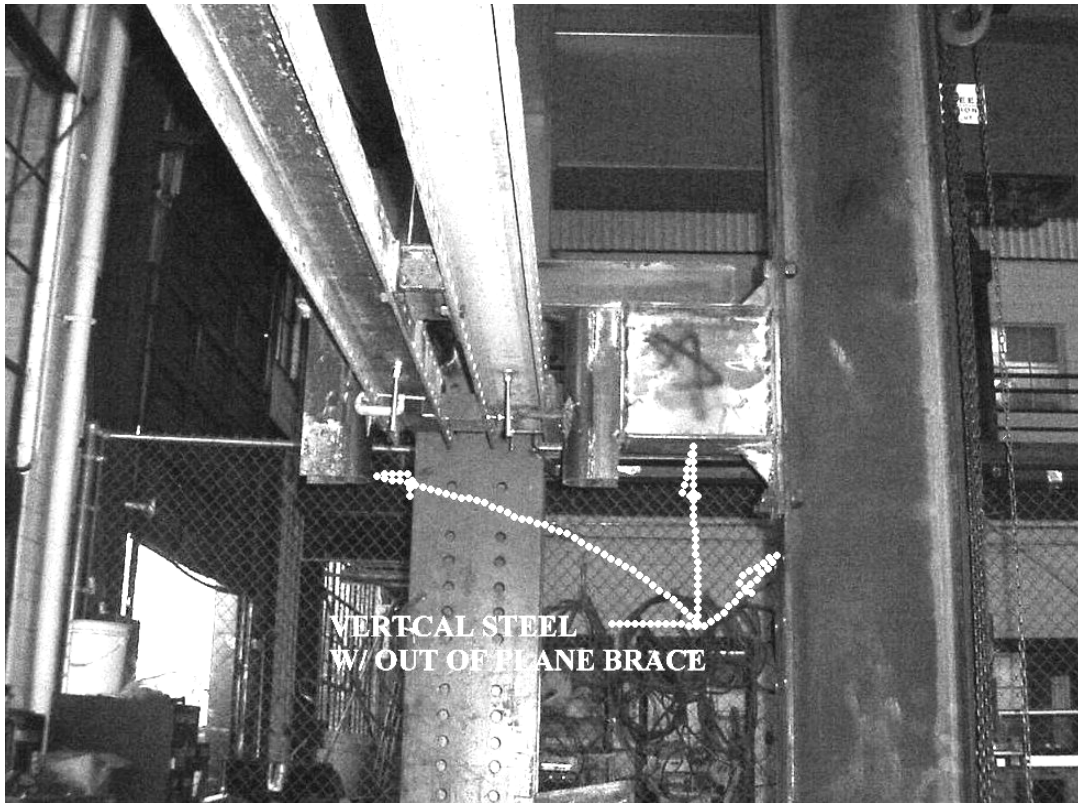
Figure C.2. Out-of-plane lateral bracing.
